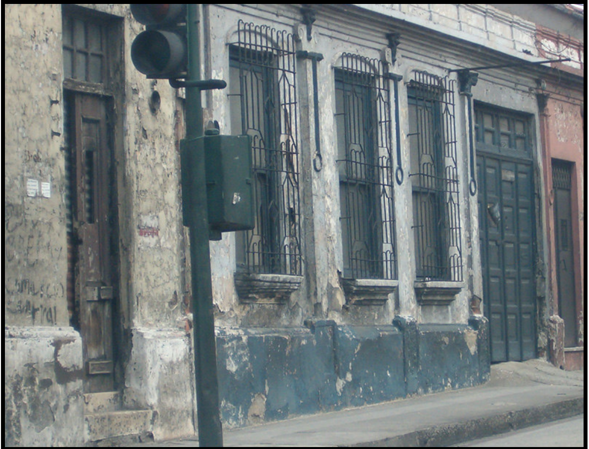
Figure 6- Zone 1: Worn Hardwood Doors and Bared Windows in Unkempt Colonial-type Houses of City Centre. House built at the turn of the 20 th century.
