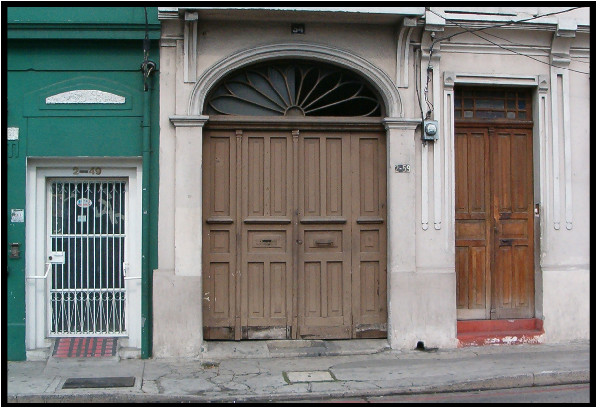
Figure 10- Zone 1: (From Left to Right) Modernized Metal Grate Door with Electric Lock on Colonial Type Home, Hard Wood Fold-out Door in Colonial Type Home, Hard Wood Entry Door in Colonial Type Home.
