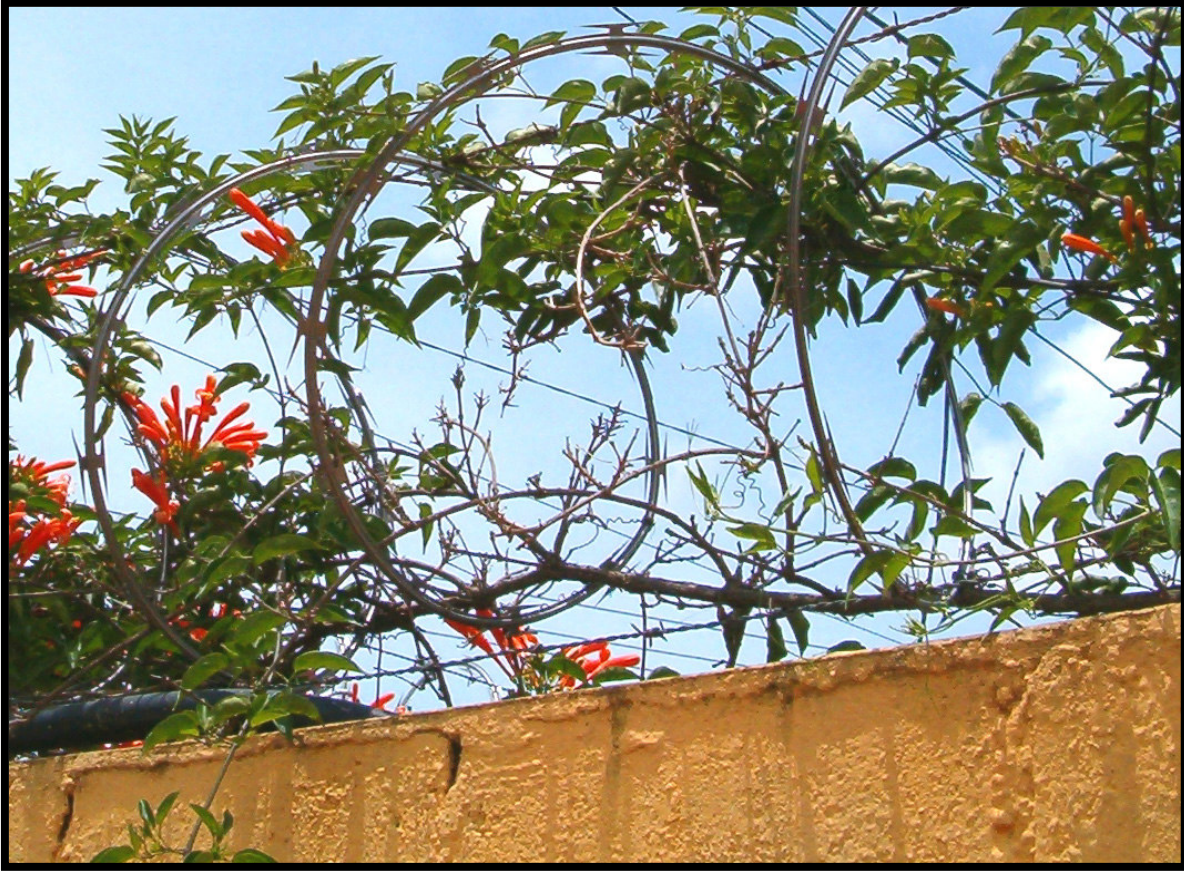
Figure 21- Zone 2: Razor and Chicken Wire Combination with Greenery Embelishment.
