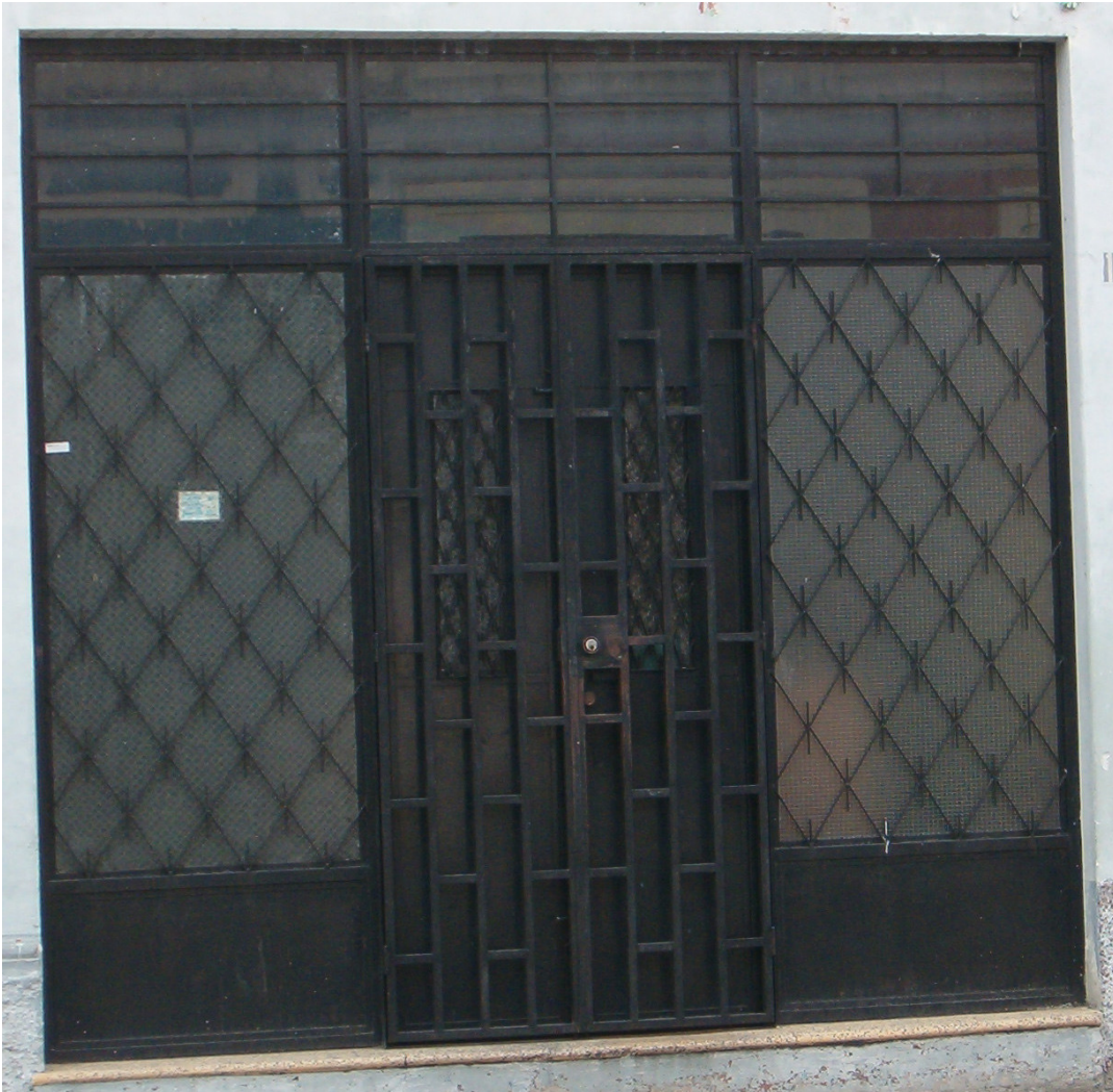
Figure 14- Zone 2: Grated Metal Entry Door with Grated Safety Glass Sides and Overhang.
