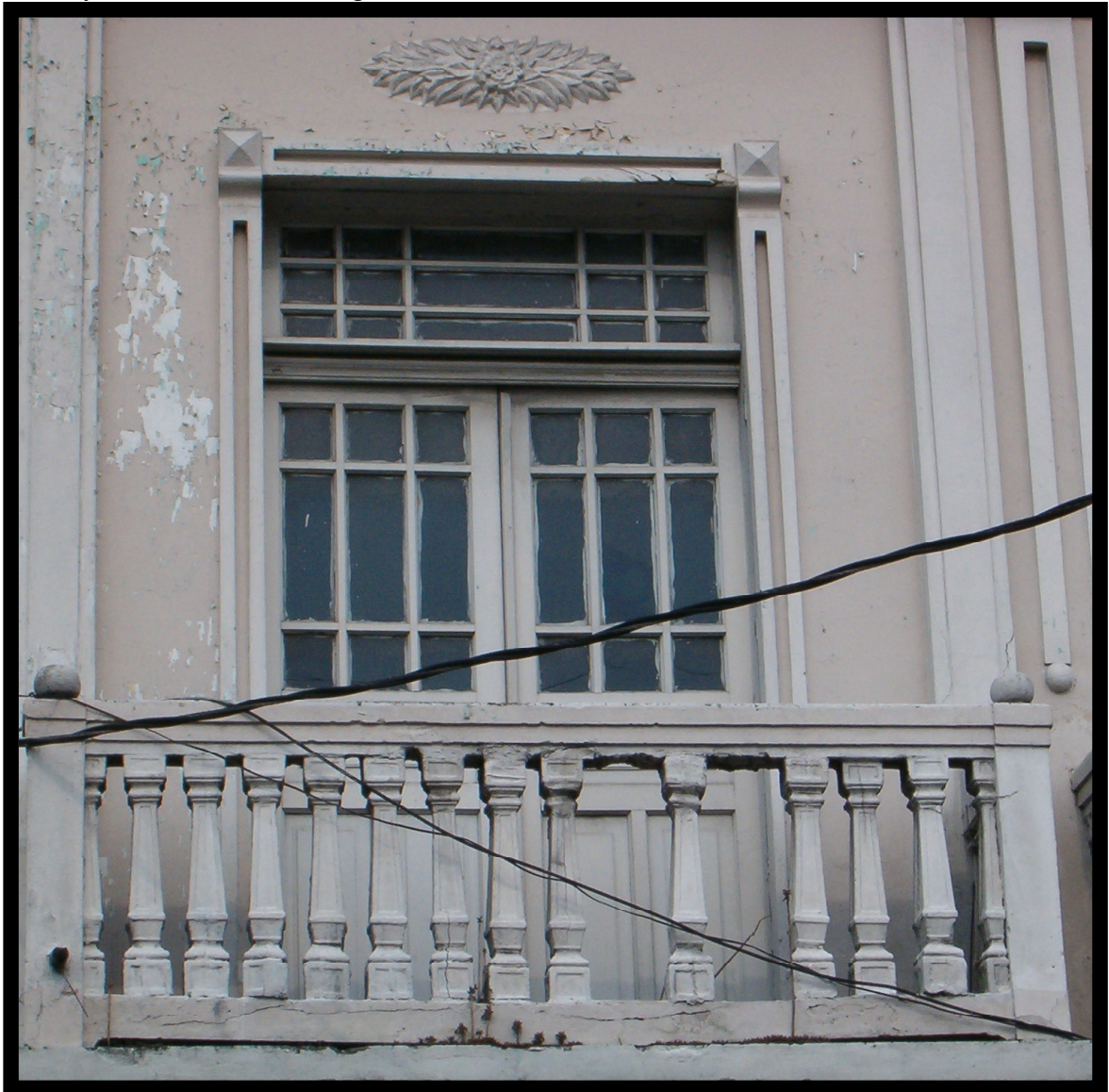
Figure 9- Zone 1: Second Floor Window with Balcony. No Security Treatment on Colonial Type Home.
