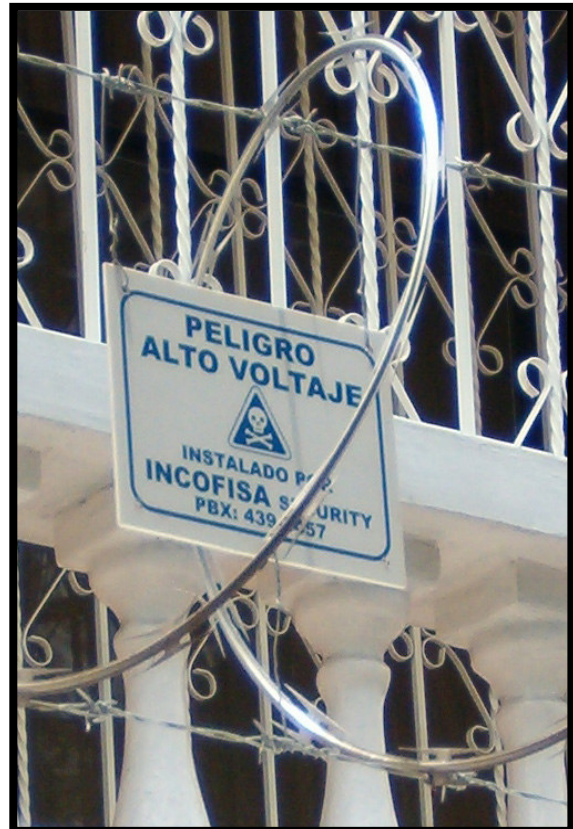
Figure 22- Zone 2: Electrified Razor and Chicken Wire Combination with Double Layered Wrought Iron Second Floor Windows.
