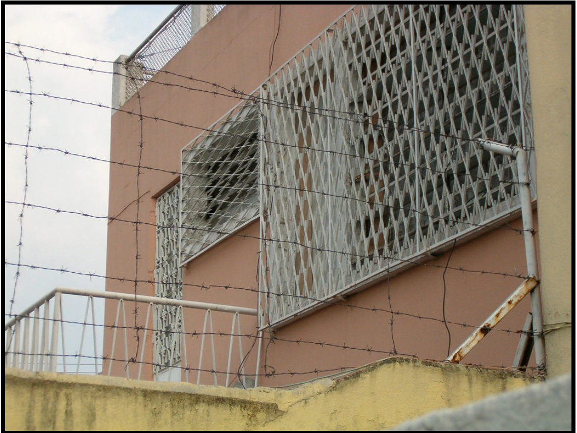
Figure 19- Zone 2: Chicken Wire and Tight Wrought Iron Window Grates on Second Floor Window and Balcony Area.
