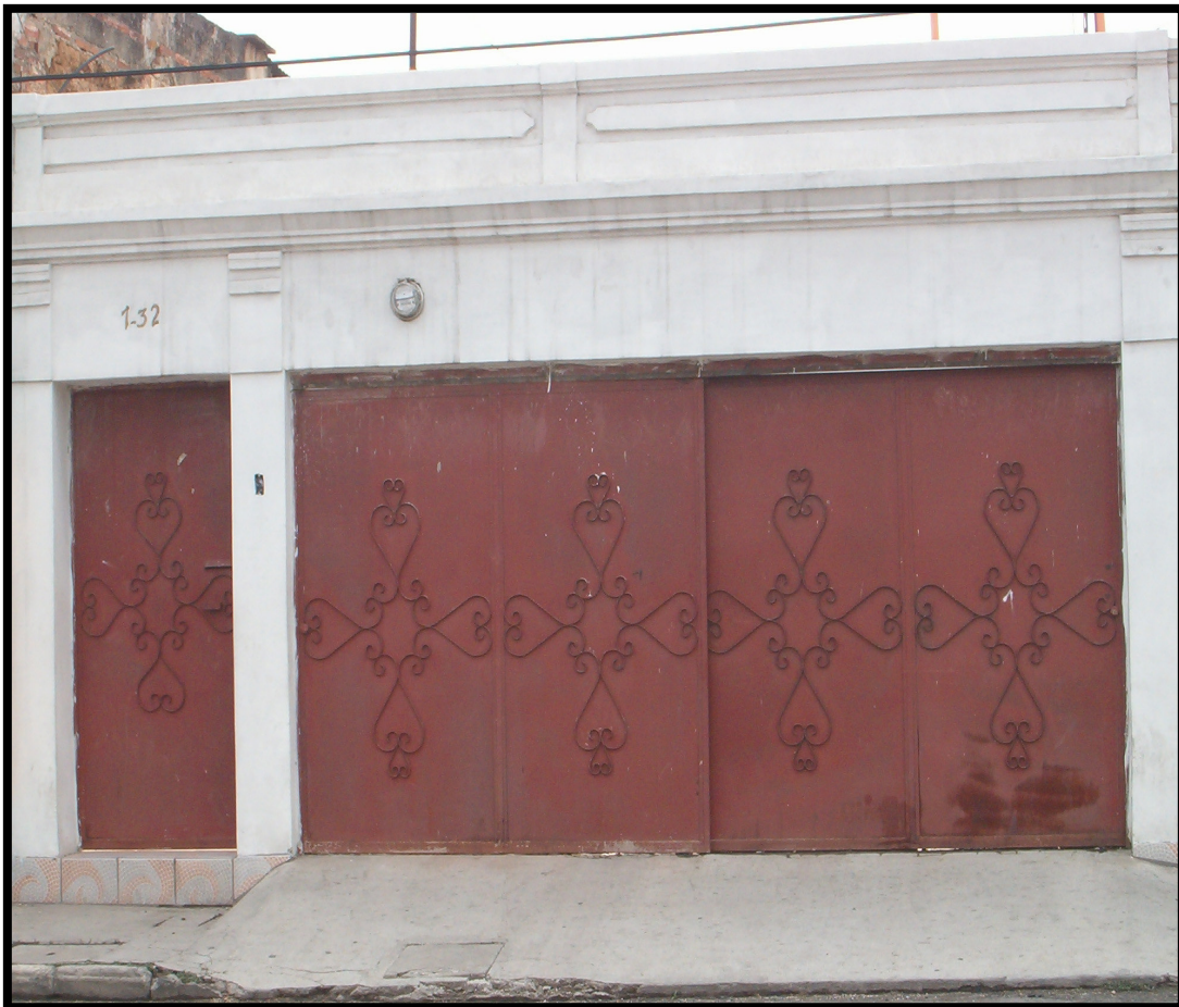
Figure 13- Zone 2: Metal Entry and Garage Doors with Wrought Iron Embellishment.
