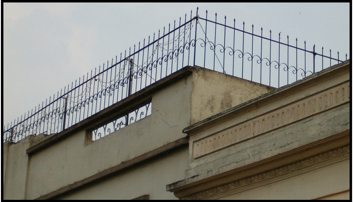
Figure 20- Zone 2: Wrought Iron Spike Fence on Second Floor Roof.
